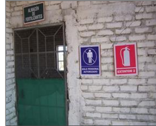
Photo of non-conformity Fire extinguisher missing.JPG
